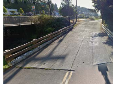
Figure A: Existing Bridge
