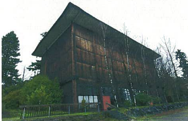
Staff photo/June Collins-McKiernan The Episcopal Church of the Redeemer (located at 6211 NE 182nd St. in Kenmore) was designed by Roland Terry, a renowned Northwest architect.
