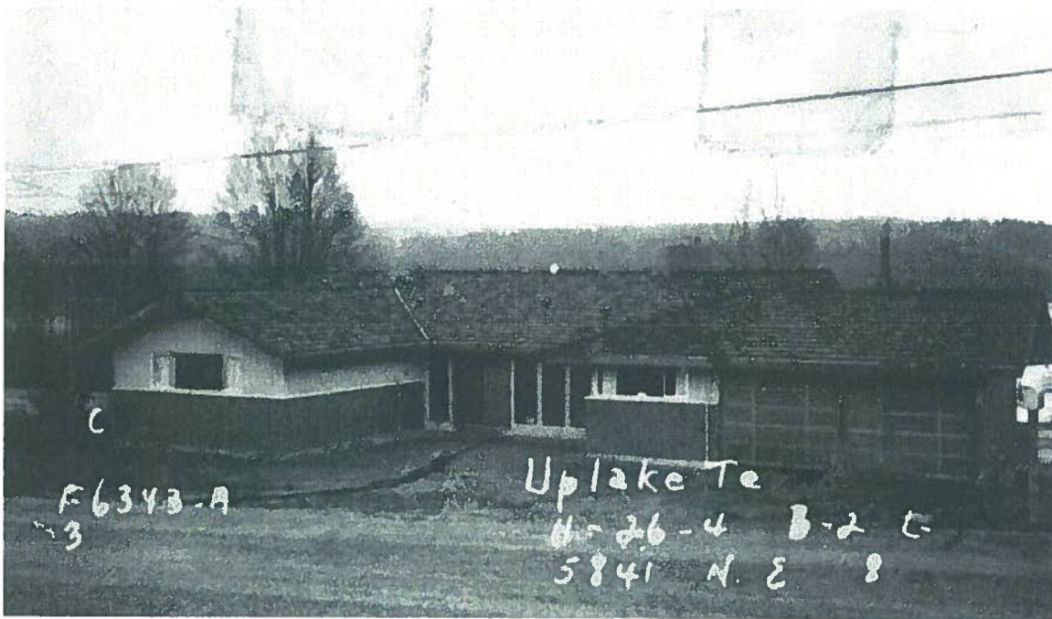
Figure 4 This Uplake Terrace house was built in 1959 and features a moderately pitched gable roof with deep eave overhangs, an integrated garage, and large picture windows on the rear (overlooking Lake Washington), all hallmarks of the Ranch style. (King County Tax Assessor)
