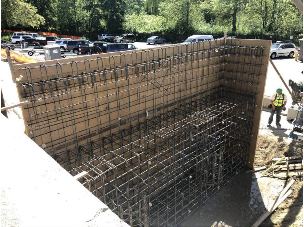
Crews continue rebar and formwork installation at the Pier 1 abutment.
