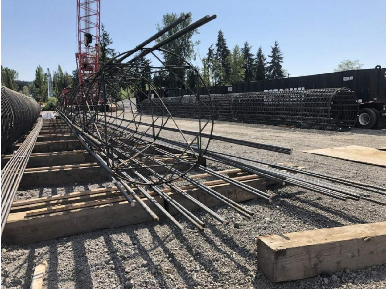
Crews assemble bridge foundation shaft rebar into circular cages ~80-110' in length.
