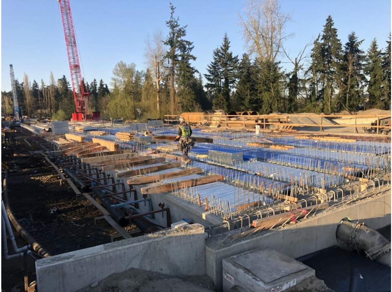
The contractor nears completion of deck formwork installation.
