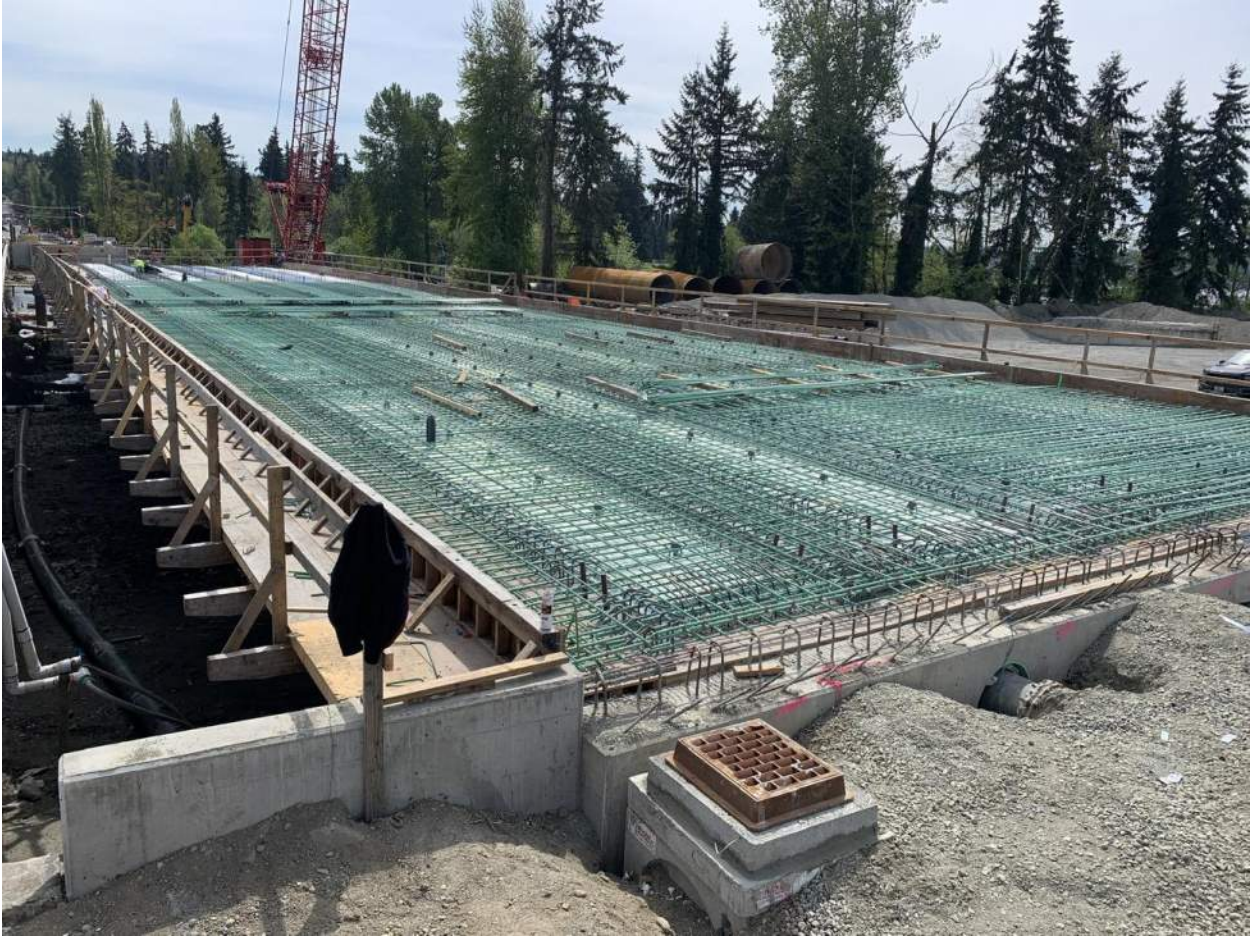
The Span 5 deck rebar installation is completed.
