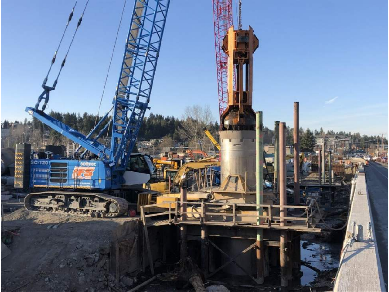
Shaft excavation at Pier 4 west column.
