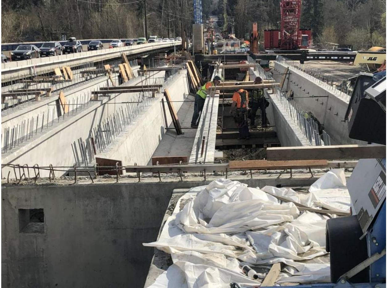
The contractor adds minor elements to the newly set bridge girders.
