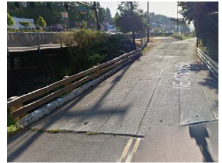
Figure A: Existing Bridge
