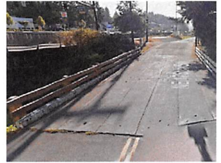
Figure A: Existing Bridge
