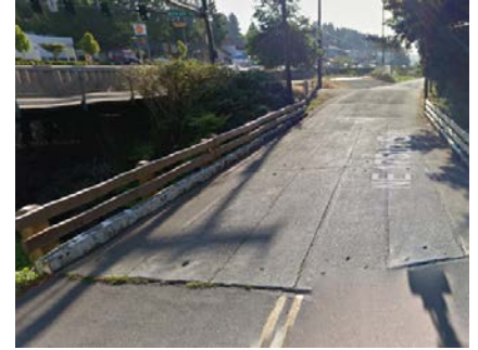
Figure A: Existing Bridge
