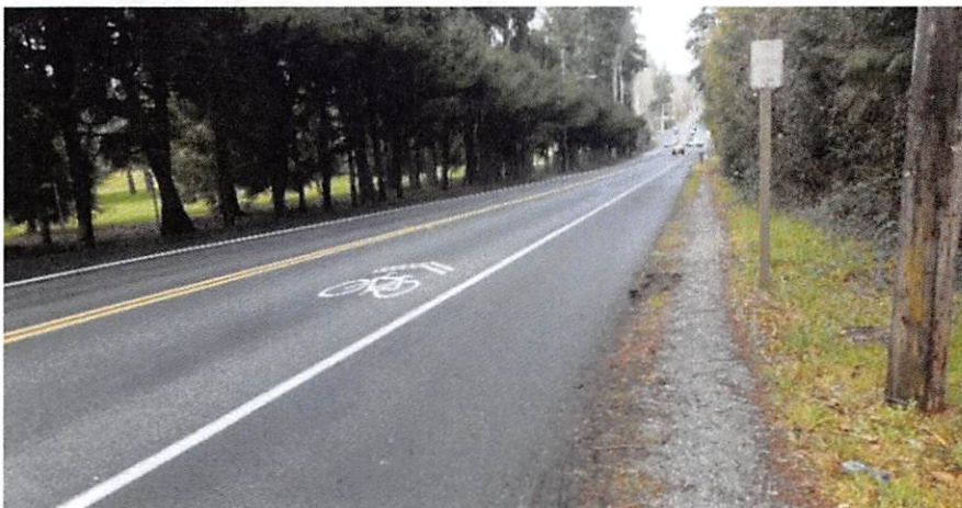
Existing Conditions on Juanita Drive
