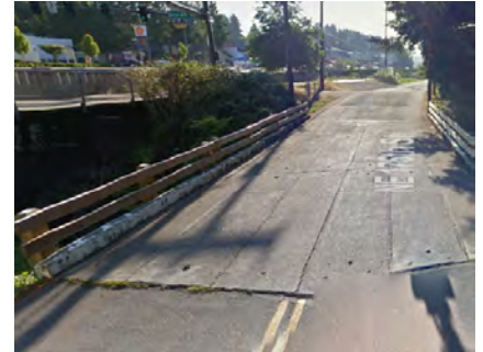
Figure A: Existing Bridge
