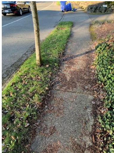
Figure 48. Juvenile subject tree that is not damaging the sidewalk and should be retained.
