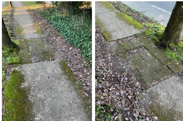
Figure 3. Pavers over the root system of Tree #102.
