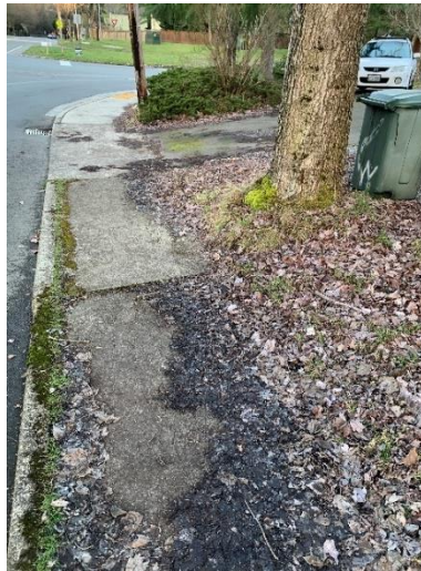
Figure 68. Minor impact to the existing sidewalk.
