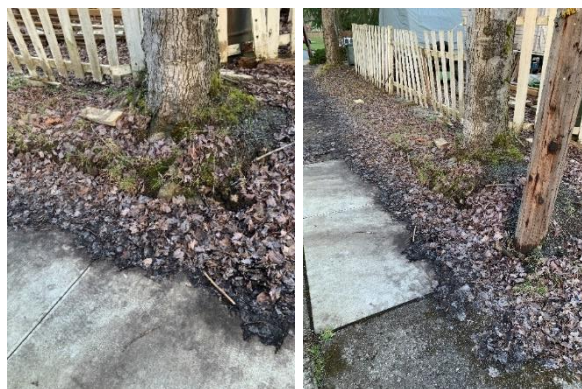
Figure 67. Minor impact to the existing sidewalk.
