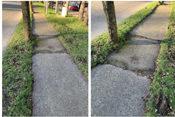
Figure 11. Trunk of Tree #110 already abutting against the sidewalk and a small planting strip.
