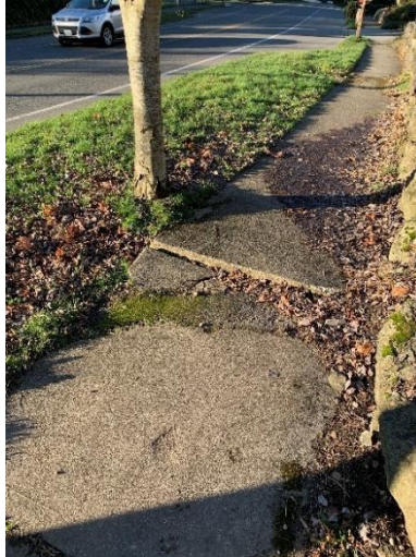
Figure 50. Bridging over the sidewalk would allow for the retention of the tree.
