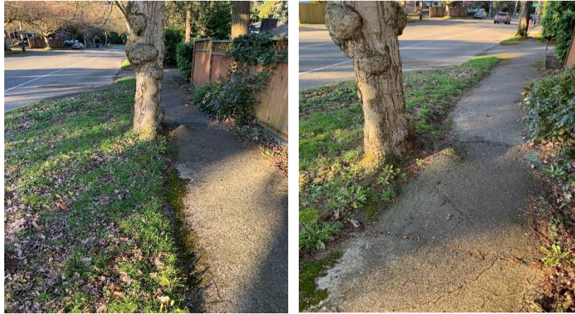
Figure 31. Multiple large galls on the stem of the tree and the significant damage to the existing sidewalk.
