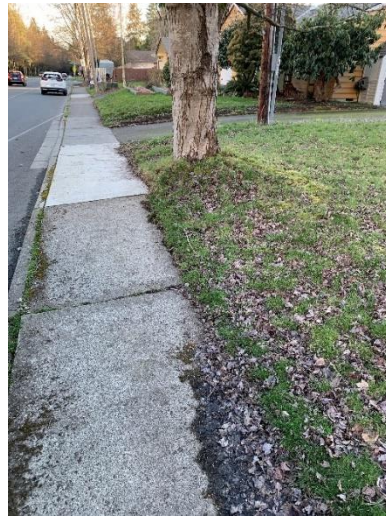
Figure 66. Minor impact to the existing sidewalk.
