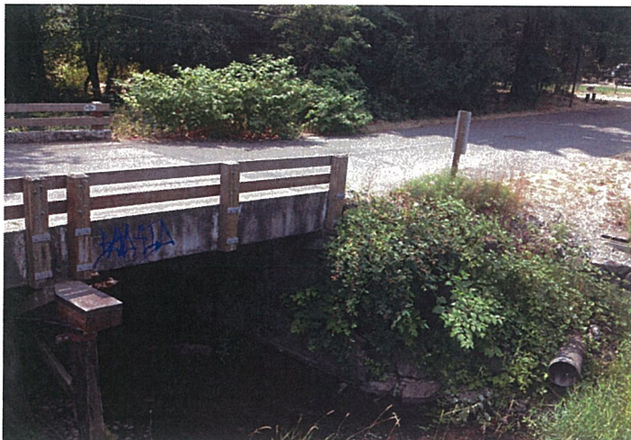
Lower Swamp Creek Bridge – Abutment
