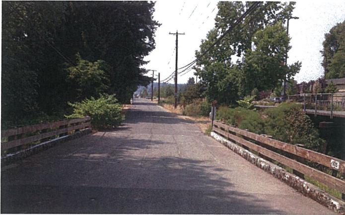
Lower Swamp Creek Bridge – Deck View
