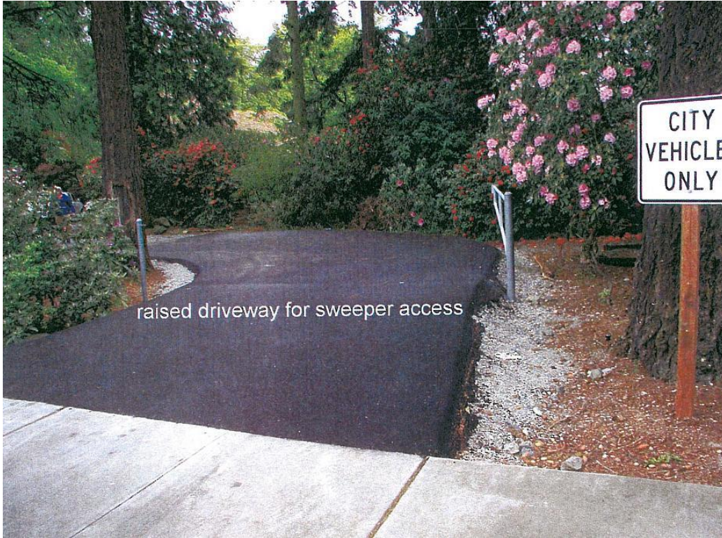
Entrance to facility from NE 170 TH ST.
