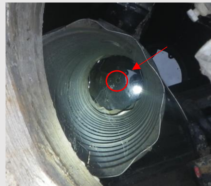
◀ The orifice plate: a plate at the bottom of the FROP-T section with a small hole (orifice) in the center. The diameter of the orifice depends on the flow volume of the system.
