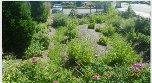
Good: this swale has healthy vegetation and a clear path for water to follow
