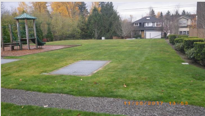
Modern residential stormwater facilities can double as recreational space for the neighborhood (Left). It usually has several solid drain lids as well as access grates for maintenance (Right).
