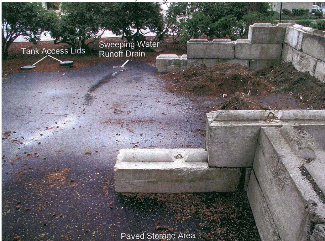
View of facility from north looking south. All surface runoff is collected in drain.
