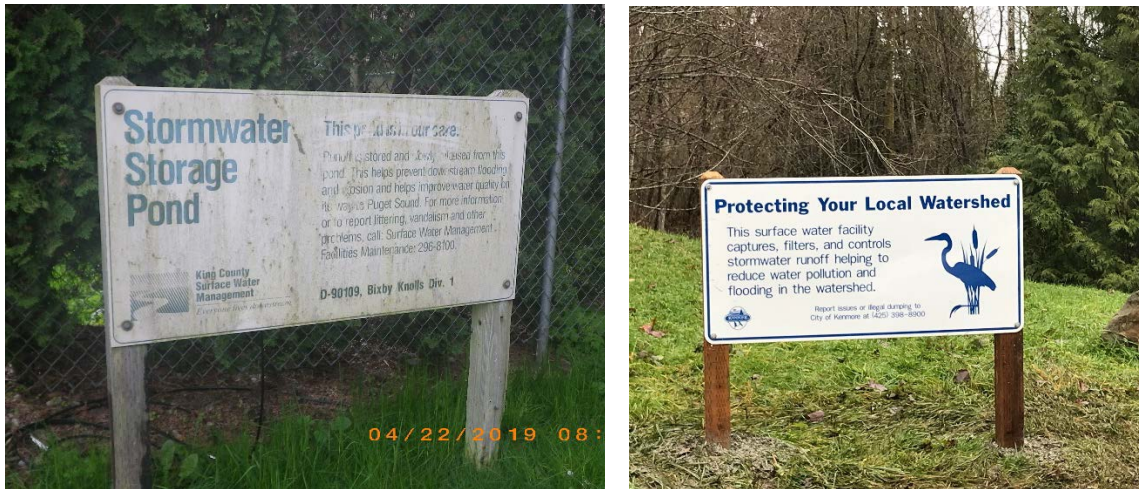
Photo: Before and After Pond Signage
